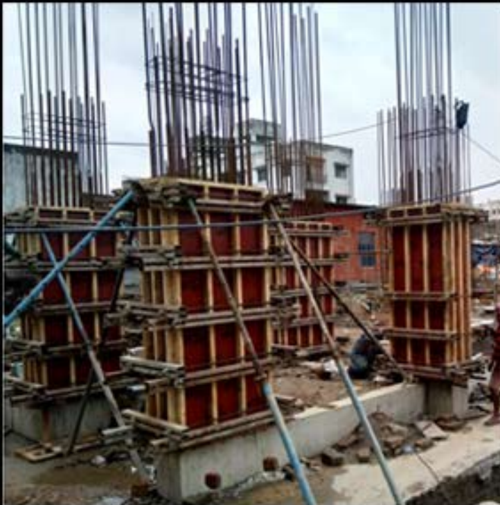
COLUMN SHUTTERING & CUSTING WORK
