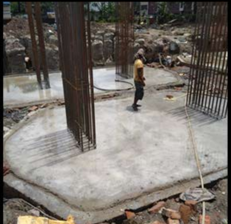
PILE CAP CUSTING WORK
