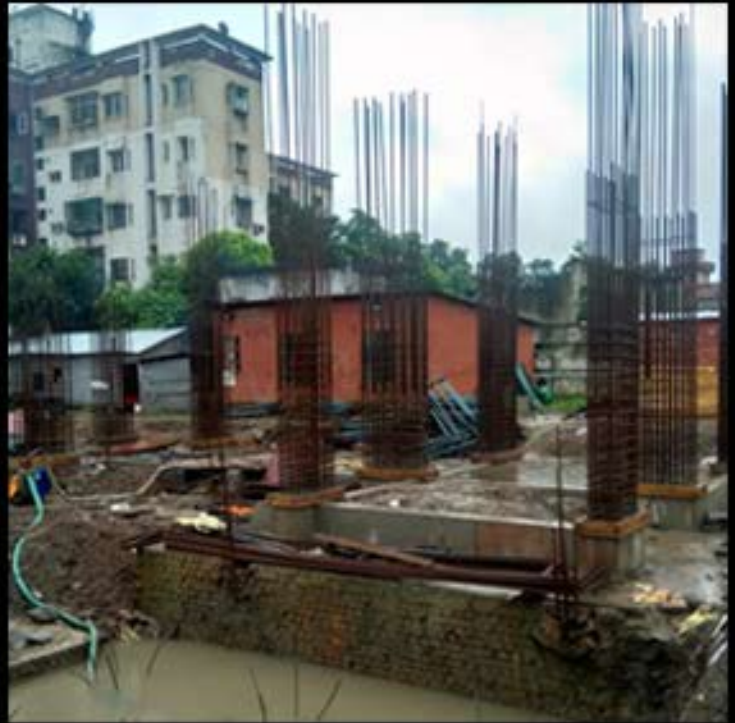
STEEL BINDING FOR COLUMN
