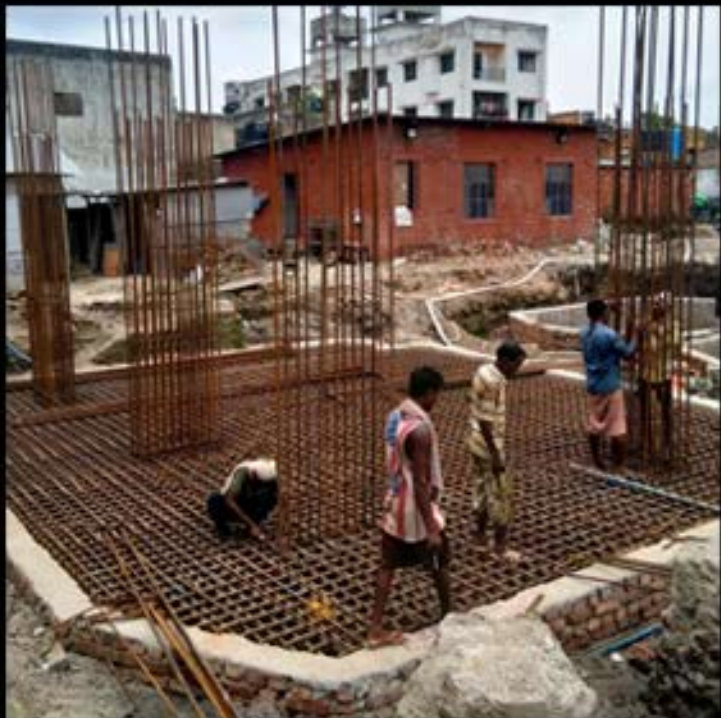
STEEL BINDING WORK
