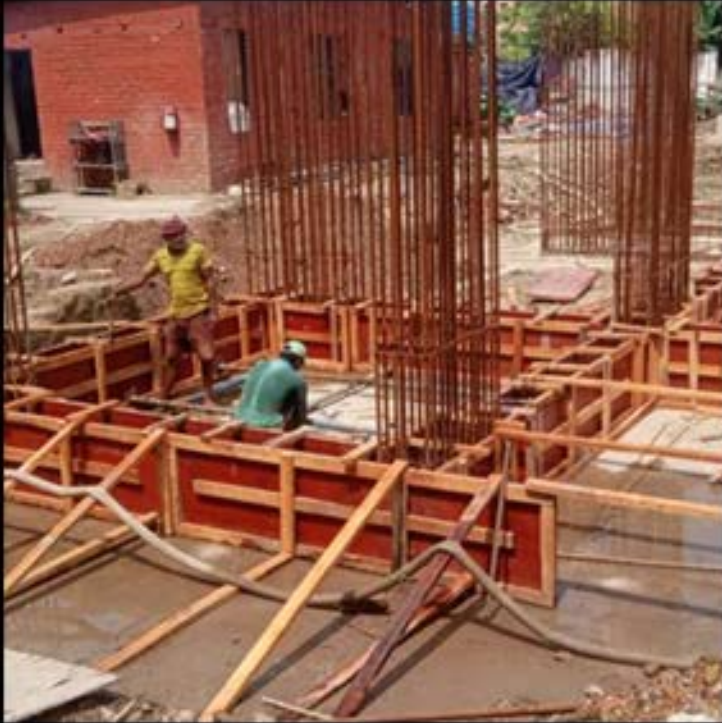
TIE BEAM SHUTTERING & CUSTING WORK
